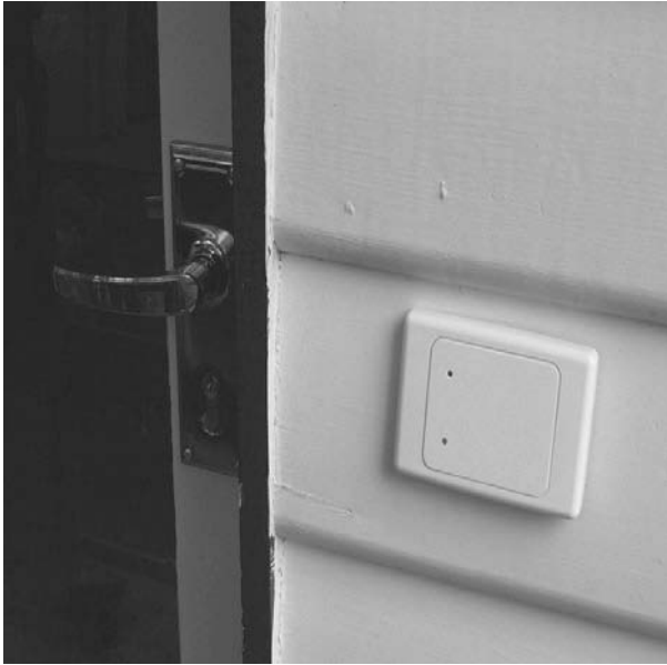
Figure 14-17. Reader mounted inside a wall plate fitted beside a door
