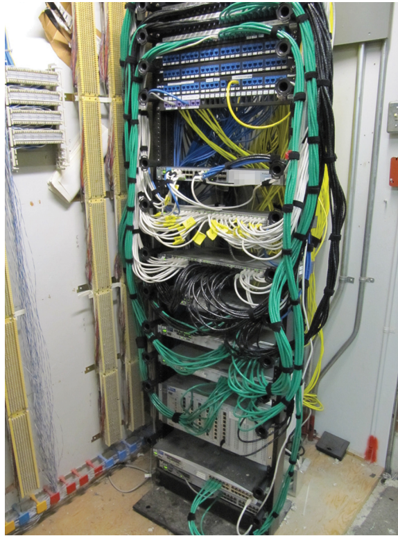
FIGURE 10.1 A typical wiring closet
