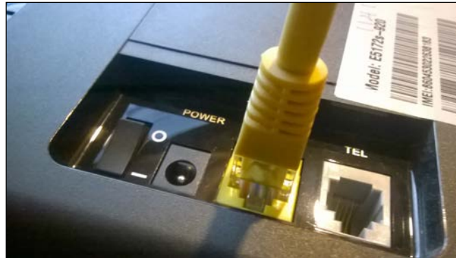
The other end of the Ethernet cable is connected to the router/switch
