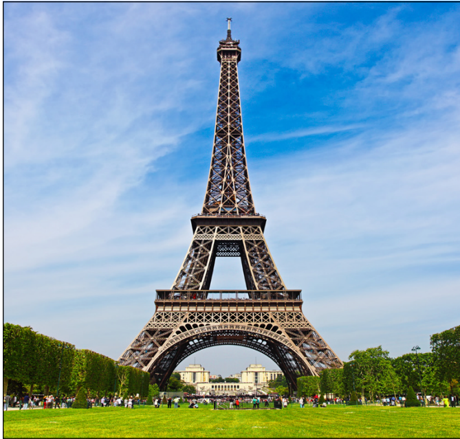
FIGURE 4-2: The Eiffel Tower is constructed of 7,300 tons of wrought iron, a low-carbon iron grade that is typically pounded into shape while hot rather than cast.
