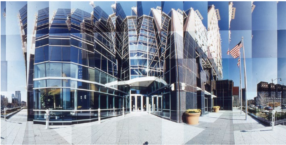
Figure 9-4. Top: OSERF Building Broad Street View, Columbus, Ohio, by Masumi Hayashi (2001). Reproduced with permission from the Estate of Masumi Hayashi.
