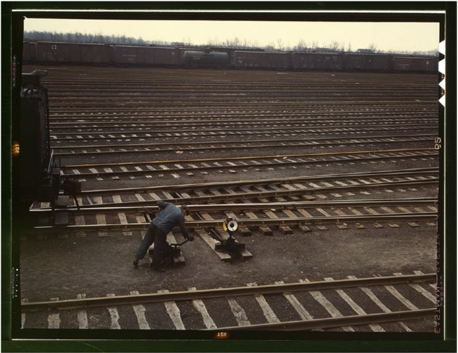
Figure 7-2. Switchman throwing a switch at the Chicago and NW Railroad Proviso yard, Chicago, IL, 1942. Photo by Jack Delano; available at the Library of Congress Farm Security Administration archives. www.loc.gov/pictures/item/fsa1992000705/PP/ .
