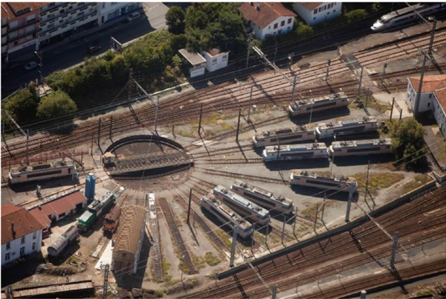
Figure 1-3. A railroad turntable. To store locomotives in a yard and to access them at any time, the central turntable would rotate to a particular set of tracks; the locomotive would drive onto the turntable, and then the turntable would rotate to another set of tracks (or would rotate 180 degrees to reverse the direction of locomotive). Source: Photograph by Jeroen Komen. https://goo.gl/PjJhgZ . Distributed under the Creative Commons License CC-BY-SA 2.0.
