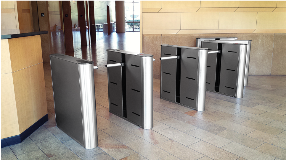
FIGURE 2.10 A turnstile can be used as a supplemental control to assist a guard or receptionist while controlling access into a protected area. PHOTO OF FASTLANE® PLUS 400 TURNSTILE COURTESY OF SMARTER SECURITY, INC.
