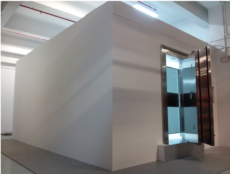
FIGURE 2.18 A vault is a room or compartment designed for the storage and safe-keeping of valuables and has a size and shape that permits entrance and movement within by one or more persons. PHOTO OF VAULT COURTESY OF INTERNATIONAL VAULT, INC.
