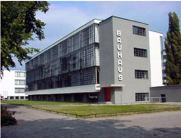
Figure 1-18. The Bauhaus building in Dessau
