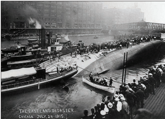
The first time the S.S. Eastland was loaded to capacity, she turned turtle next to her dock on the Chicago River. More than 800 people drowned. It turns out that the weight of her extra lifeboats was a contributing factor in the disaster.
