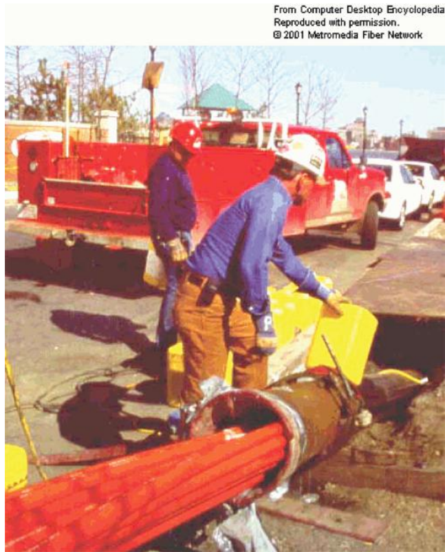
FIGURE 7.12 Burying fiber optic cable bundles (Courtesy of Computer Language Co. Inc.).
