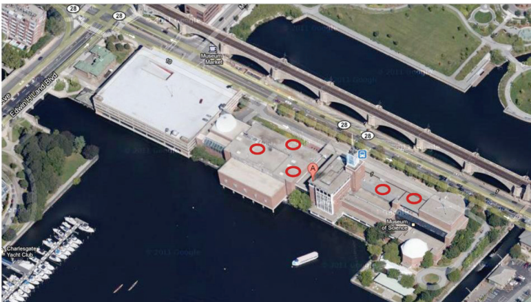
FIGURE 10.5 Red circles show location of anemometers on rooftop of Museum of Science, Boston, Massachusetts.
