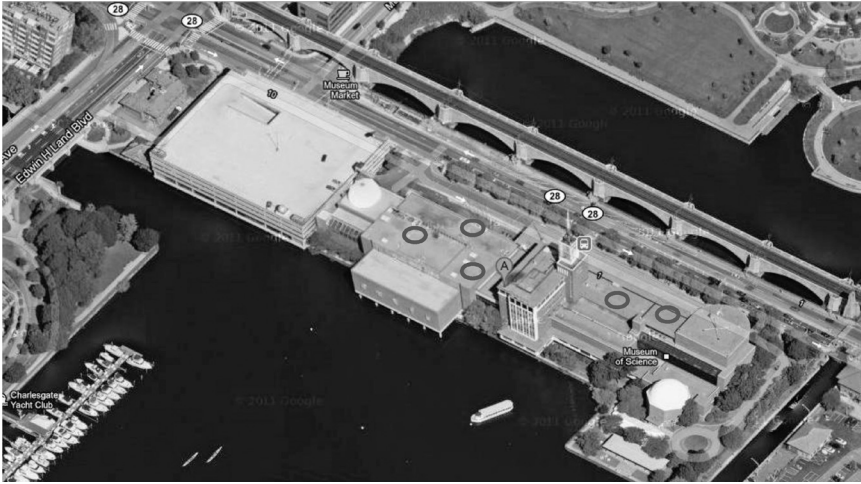
FIGURE 10.5 (See color insert.) Red circles show location of anemometers on rooftop of Museum of Science, Boston, Massachusetts.
